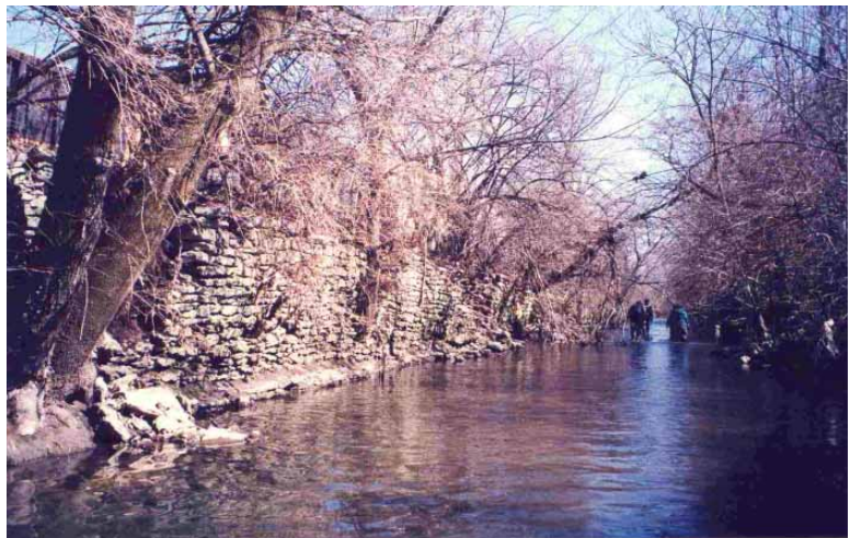
An historic dry-laid stone wall testifies to the long and continuing interrelationship between Lexington and Town Branch.
